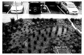
Bioretention areas function as soil and plantbased filtration devices that remove pollutants through a variety of physical, biological, and chemical treatment processes. These facilities normally consist of a grass buffer strip, sand bed, ponding area, organic layer or mulch layer, planting soil, and plants.
