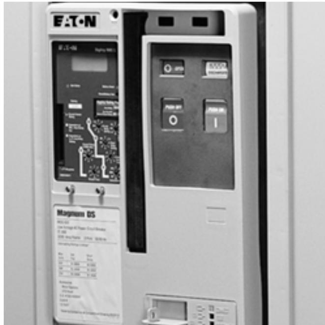
*Through-the-Door Design for Human Interface with the Breaker Compartment Door Closed*
